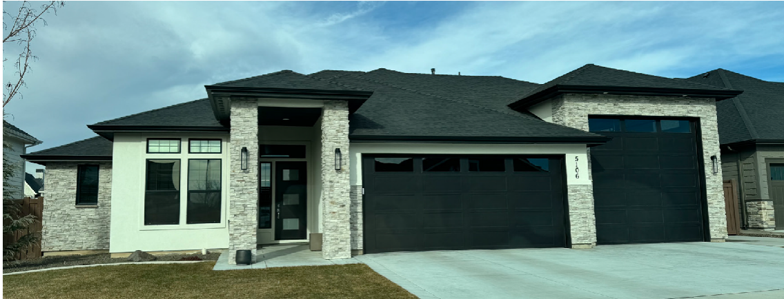
Example of too much roof facing the street (not permitted)
