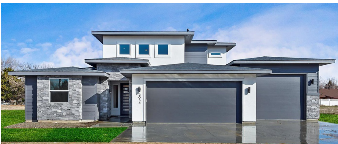
Hipped roofs will be permissible where the roof has a low slope and multiple roof breaks
